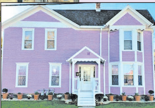
26 Elm Street won first place in the multi-family category of the 2024 Home Beautification Contest with siding repairs, new paint, landscaping, replaced gutters, and the demolition and rebuilding of the porch. (Submitted photos)
