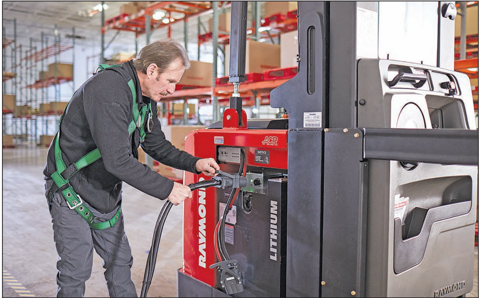
A Raymond employee charges a lithium-ion battery. The Raymond Corporation finalized its deployment of a full-scale battery energy storage system, solar microgrid array and warehouse energy management system at its distribution warehouse in Greene with the additional unveiling of a new battery manufacturing facility in Kirkwood, New York, that will build lithium-ion batteries. (Submitted photo)
